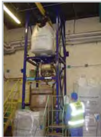
3. Traversing bag into position.
