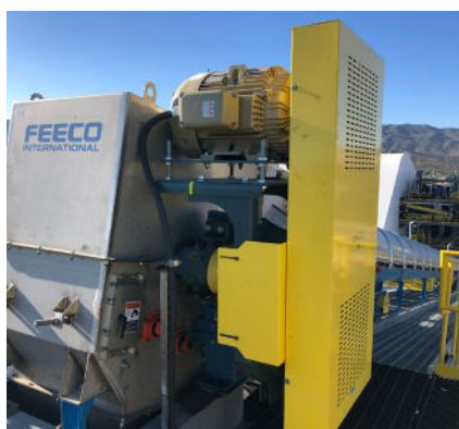
Conveyor head section (guarding and walkway visible)
