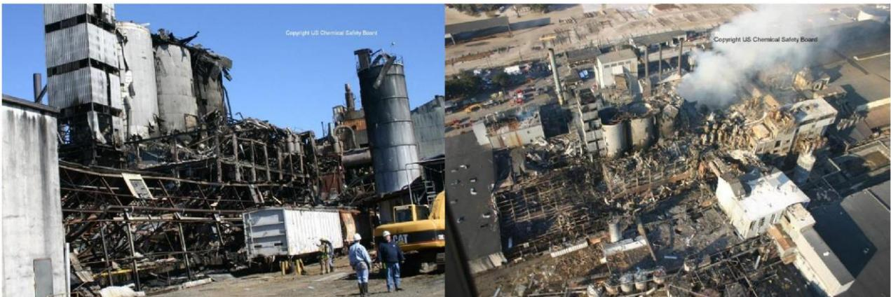
Secondary explosions may be avoided by good housekeeping and appropriate process control, stopping dust from leaking, implementing good cleaning regimes and keeping the factory clear of dust.
