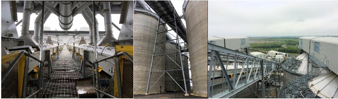
As will be noted, and expected, each of the main storage silos are fitted with explosion panels and slam-shut valves to protect the silos and their contents. Once having been extracted at a controlled rate from the main storage silos the biomass fuel pellets are, once again, transported to the intermediate silos by a twin, air supported, belt conveying system.
