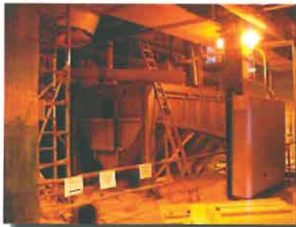
Above: the new hot pit at Barrow-on-Soar, under construction by Fairport.
