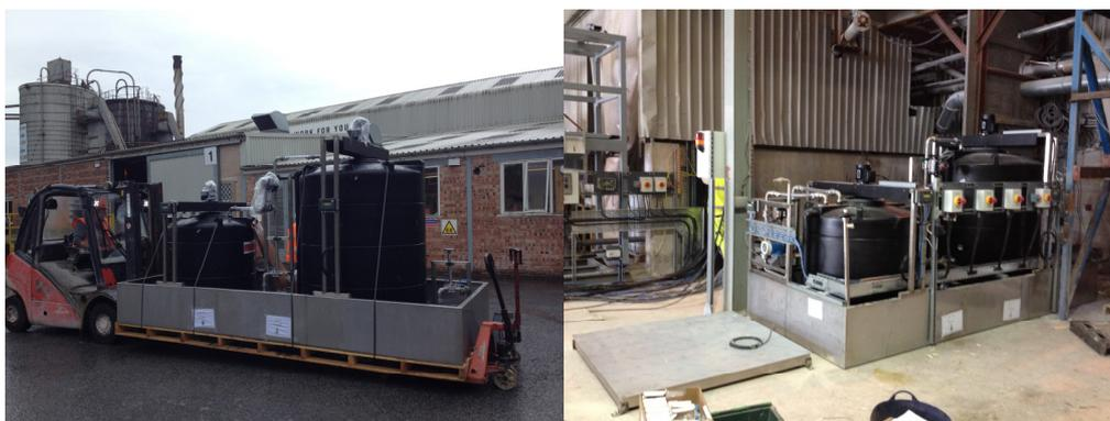
The complete dosing skid was manufactured in a standalone bund to enable ease of installation and testing and prewiring of major components. Tank levels were monitored by means of load cells to cross check dosing rates and continuously monitor levels to allow complete automation and a effectively provide a continuous dosing unit from a batch make up system.
