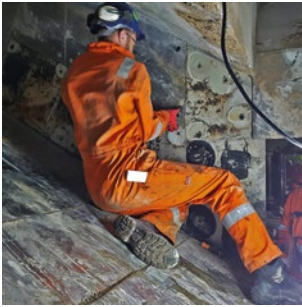
Removal of worn liner plates
